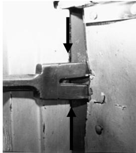
This involves working the **FORK** of the halligan into the **GAP** between the door and jamb. The arch of the **FORK** should be even with the inside edge of the door
