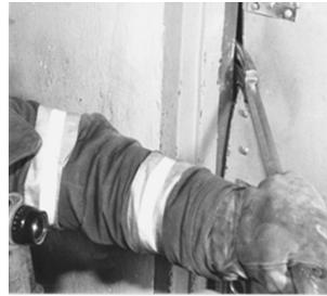
When the halligan is "**SET**" force is applied to the tool creating leverage against the door. Both firefighters should position themselves facing the door and push in sharply for maximum force
